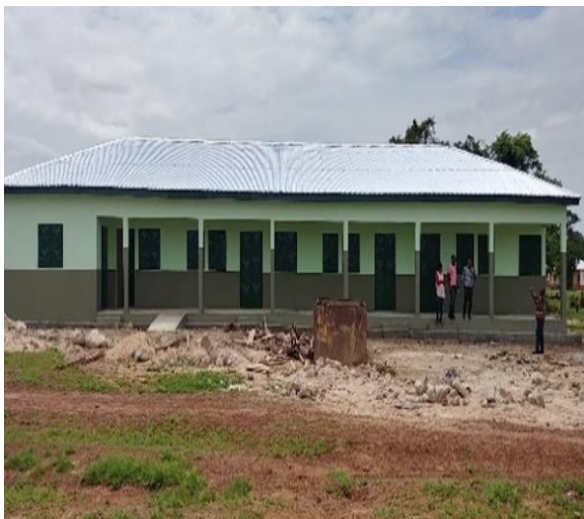
PIC 3; 3unit classroom block at Naro
